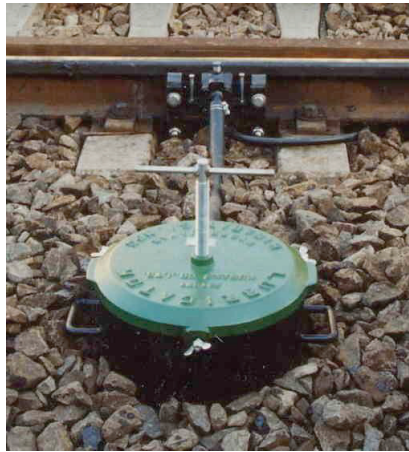
Fig. 2.12 Wayside lubricant system
