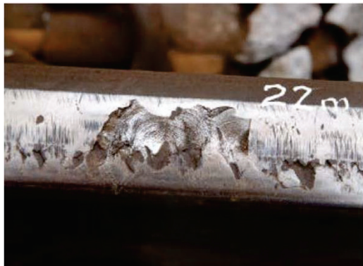
Fig. 1.35 Rail crown surface at the accident point (Flaking from horizontal defect) [22]
