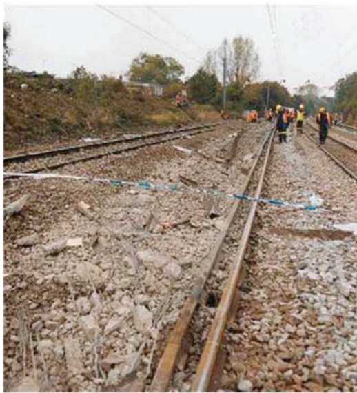
Fig. 1.29 High rail smashed in pieces at the derailment accident [22]
