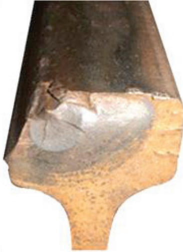
Fig. 1.8 Vertical defect in rail head
